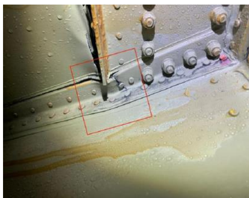
Figure 1: The left hand inboard AFT stiffener (ARM-PANEL-#6 BULKHEAD, PN: 13A01427-022) of the number 6 bulkhead has been cracked
