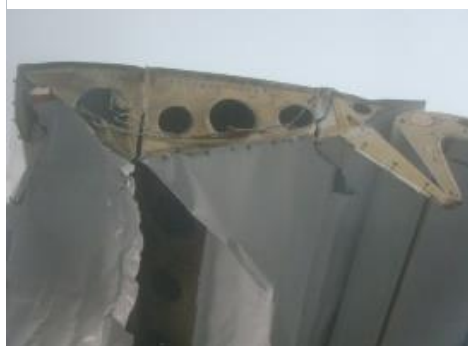
Figure 6 LH Wing (RIB NO. 28) Damage
